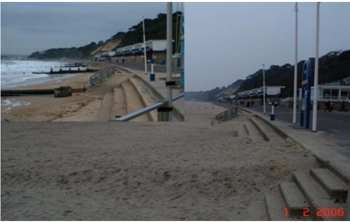
Figure 3: Before and after: beach nourishment using dredged sediment from the deepening of the navigation channel in Poole Harbor.
