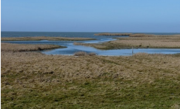
Figure 2: The natural foreshore in Lake IJssel, protecting the dikes against high wave action. The dredged material of nearby harbour maintenance was used.
