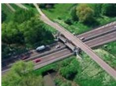
The photo shows the structure at the intersection of the Dief dike and A2. When a flood event occurs, a barrier closes down the A2 to allow the Dief dike to carry out its compartmentalisation function.
